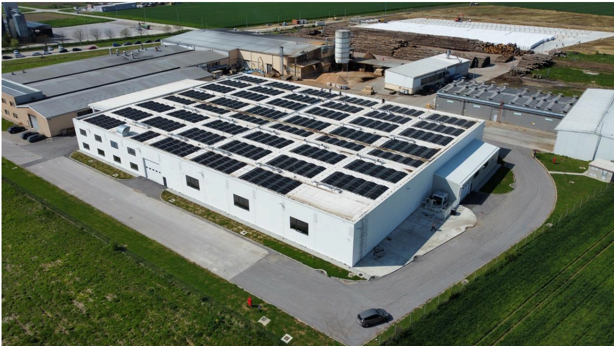
Veneer splicing factory with solar panels
